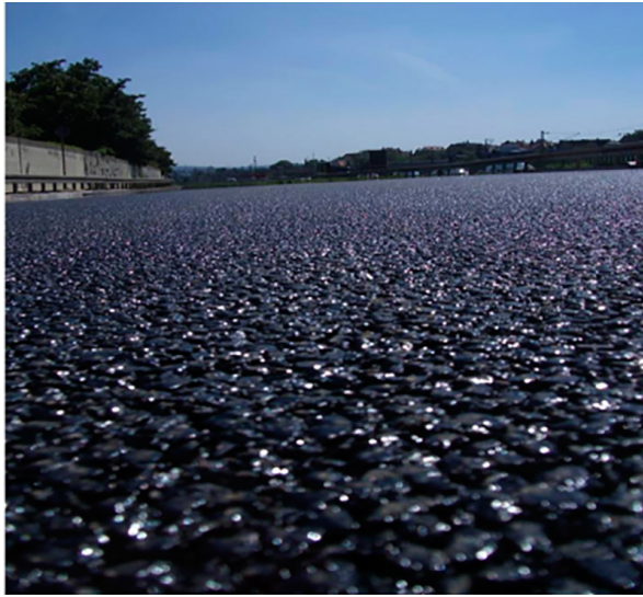
Figure 3 and 4, Noise Reducing SMA, Surface Texture
